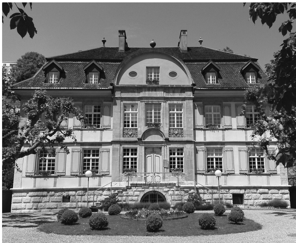
View of Valltravers' House «Rockhall» in Bienne
